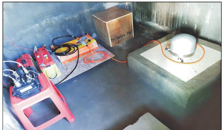
Installation of new broadband seismograph (BBS) at Rain Forest Research Institute (RFRI) campus, Jorhat, Assam.
